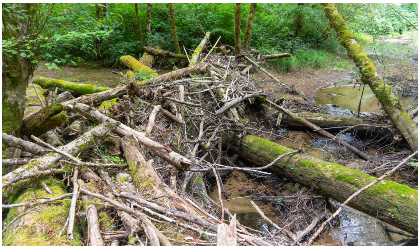
Figure 7.9. Large wood placement project in Elk Creek, completed by Coos Watershed Association.
